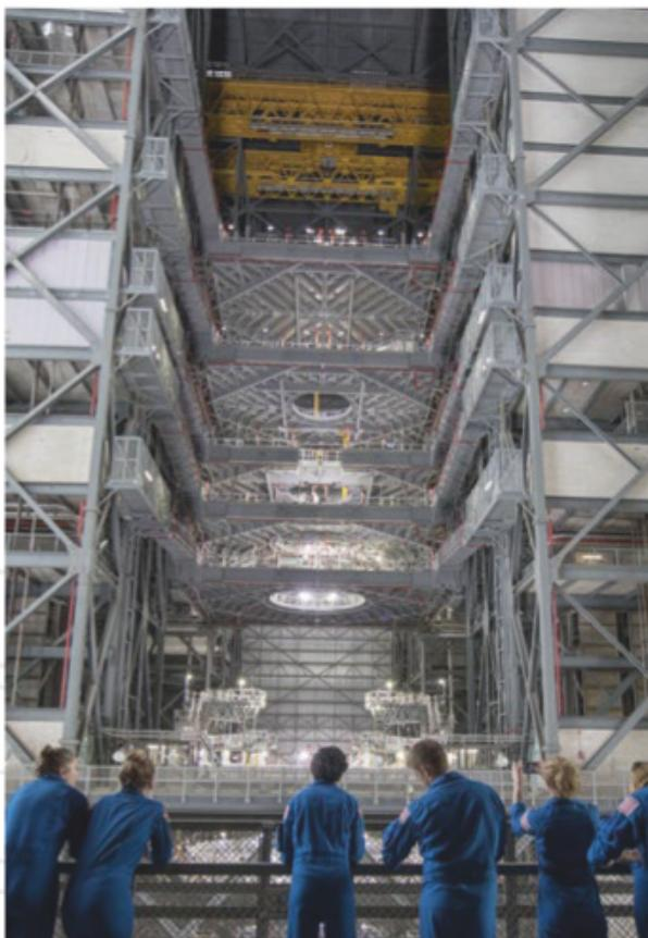
Currently, VAB is ready to house NASA's upcoming Moon rocket, SLS. Although the rocket becomes the world's largest and will measure 111 meters in height, there is plenty of space under the 160 meter high roof. The building can accommodate a total of four assembled SLS rockets.
